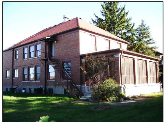
Cantigny Cottage, 2010. Photo courtesy of former resident Lou Williams.
